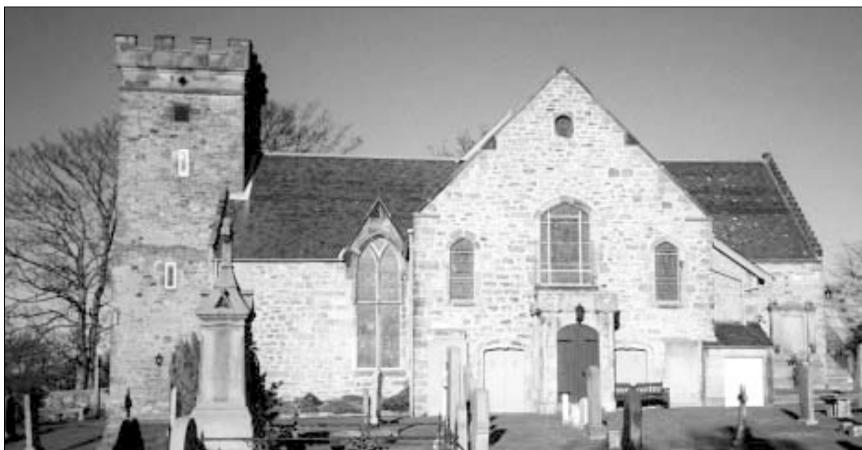
Figure 2 Cramond church. This has a fifteenth century tower and a seventeenth century transept and nave.
