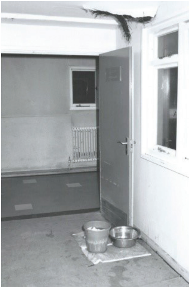
Figure 6 Damage to the wards after a flood and because of ageing facilities. Personal photograph
